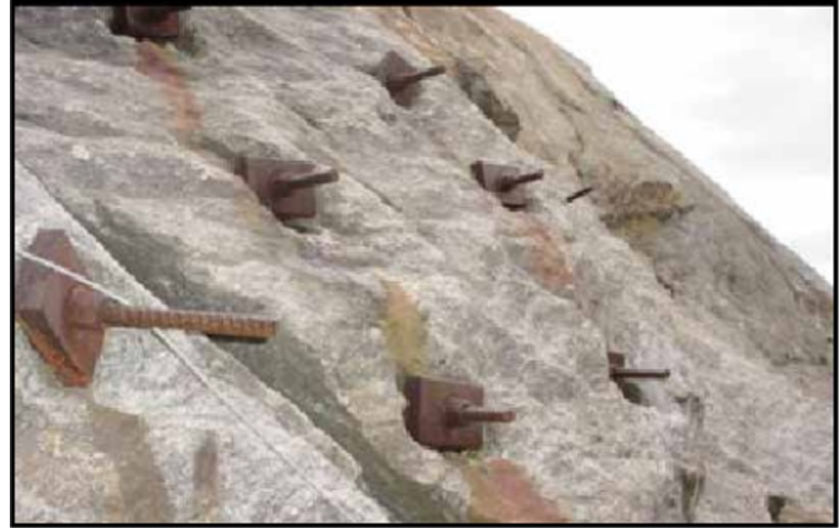
Fig. 3.30: Rock anchors
